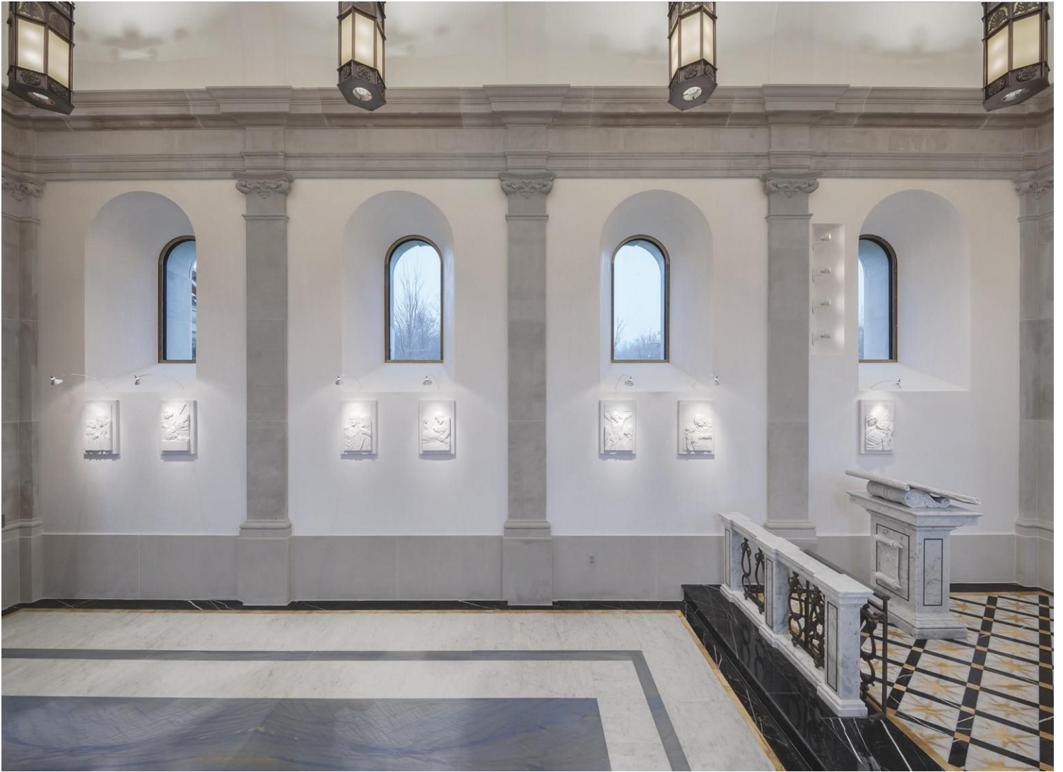
Indiana Limestone, procured from Rugo Stone of Lorton, VA and Bybee Stone Company of Ellettsville, IN, trims the windows, doors and eaves.
